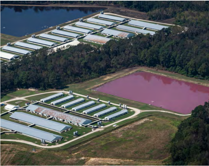
An aerial view of buildings and waste holding ponds at a concentrated animal feeding operation (CAFO) in North Carolina.
