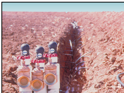
Figure 7. Laying subsurface drip (a) and the pump that maintains the flow of water through the system (b).
